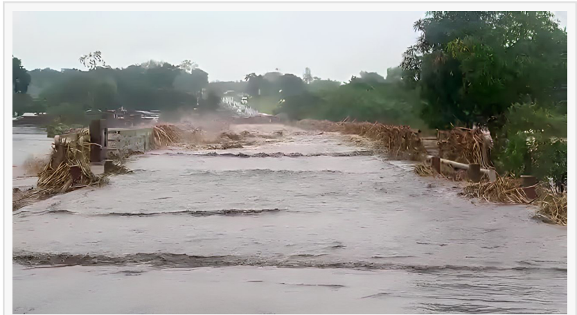
Bridge on the Mulanje-Thyolo Road
