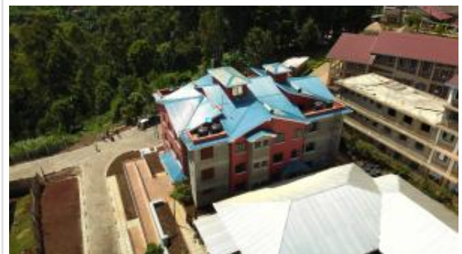
Aerial View of New Residence Hall at Clive Irvine College.
